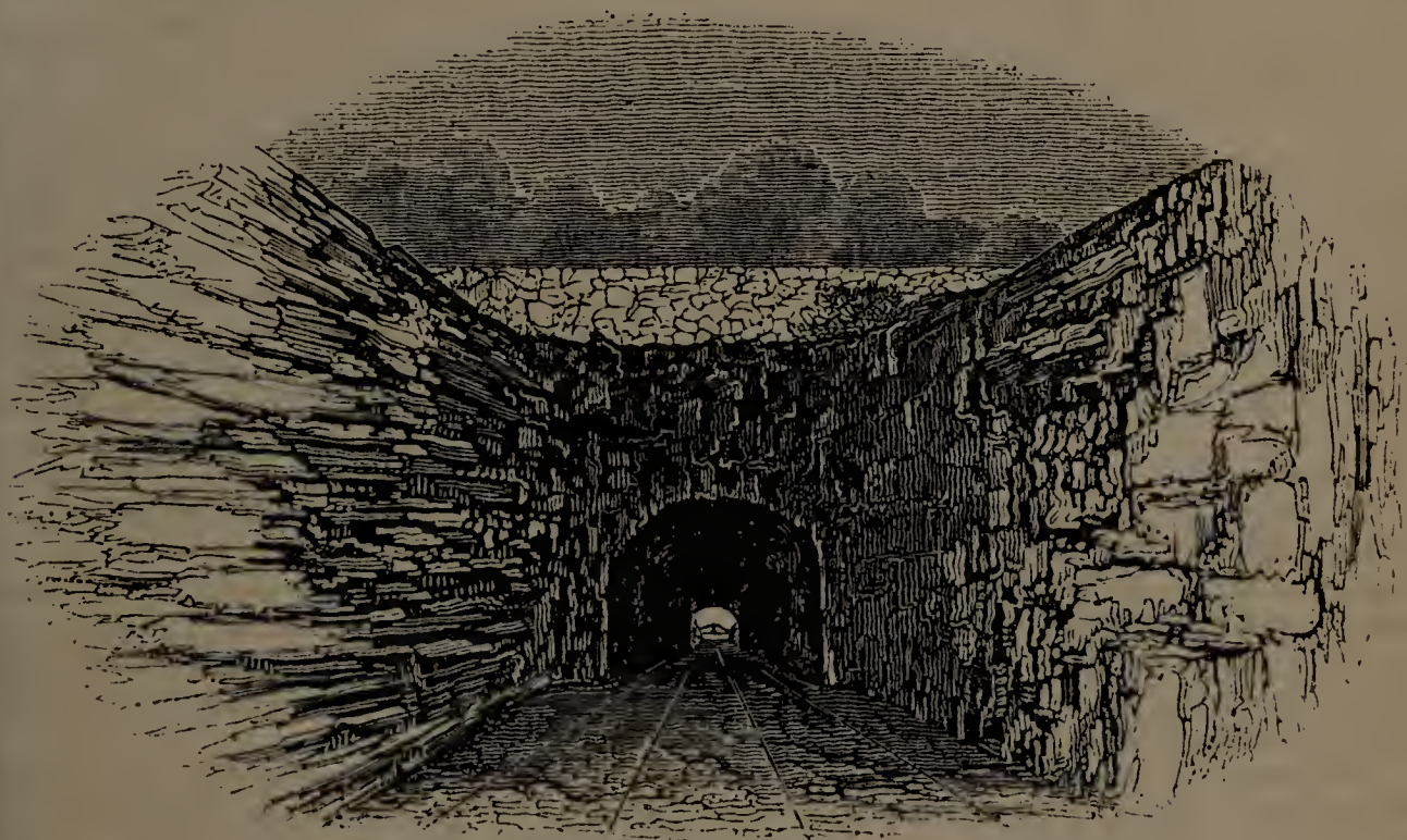
Northern view of Harlem Tunnel.
